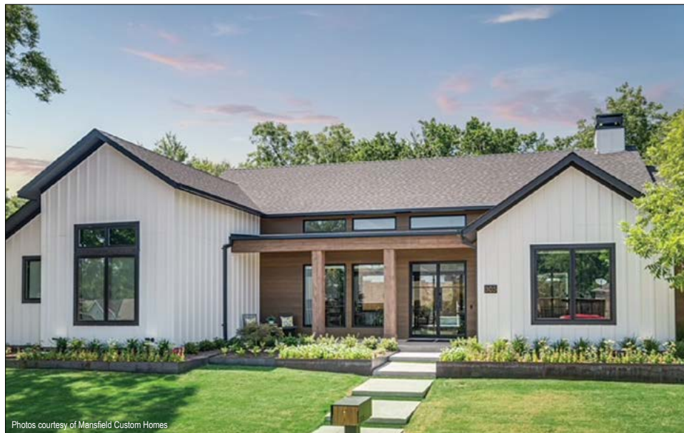
Photos courtesy of Mansfield Custom Homes
